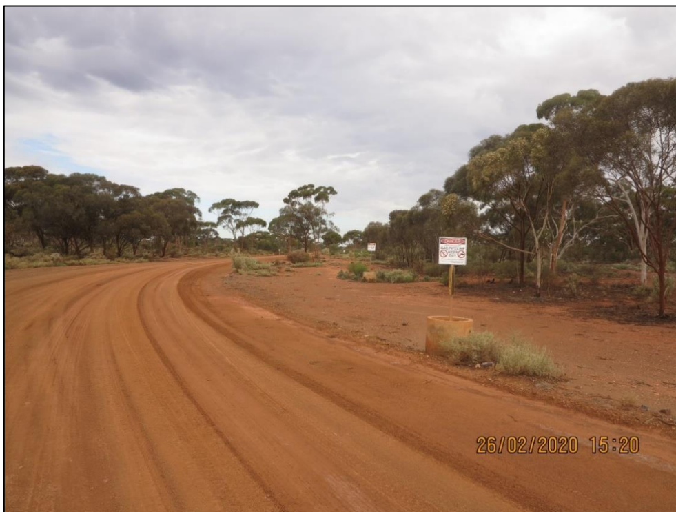
Figure 2: Carriageway looking east, showing road condition
