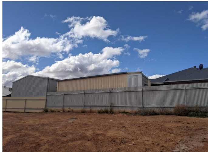
Image 4: Rear fence supported by retaining wall above natural ground level
