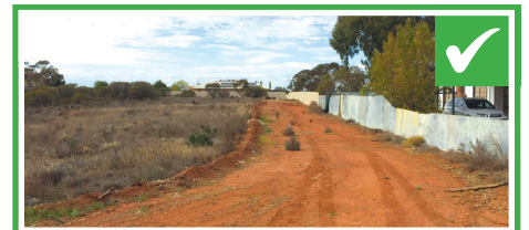
Firebreak installed on land (5,001 m 2 or greater) showing good, wide, clear boundary firebreak
